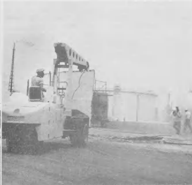
LIKE A dentist pulling teeth, this specialized vehicle jerks out storage tank sections with speed and ease. The steel sections are slated for the scrap pile.
